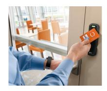
When a door equipped with an access control reader allows free egress using normal operation of the hardware, it is not typically considered one of the special locking arrangements.
