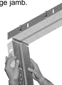
Sleeve the hinge jamb over the wall. Bring the header down tight, interlocking the stop in the alignment tab. **Try to place the hinge jamb close to the stud to assure more room for adjustment in future steps.**
